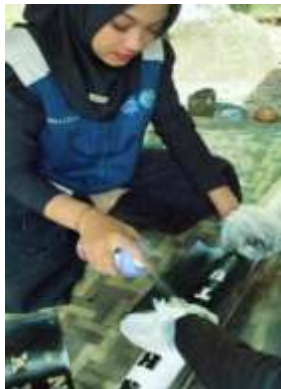
Gambar 3. Proses pengecatan pipa
