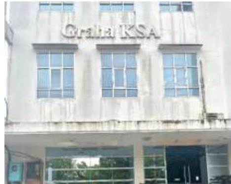
Gambar 5 Kantor PT KSA Site Samarinda
